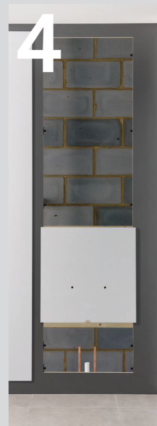
04 Drill or cut out for sanitaryware.
