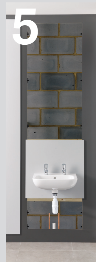
05 Mount combined panel, sanitaryware and brassware onto flashgaps before completing pipework.
