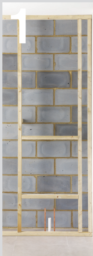
01 Install timber-frame (supplied by others).
