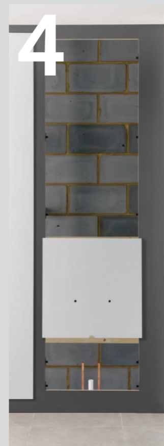
04 Drill or cut out for sanitaryware.
