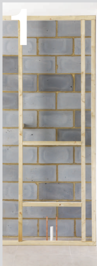
01 Install timber-frame (supplied by others).
